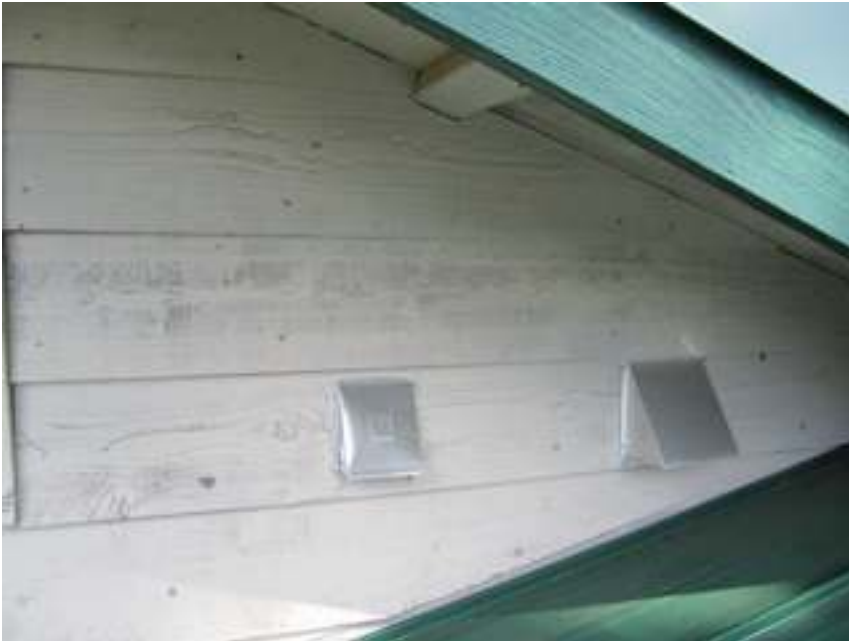
typical kitchen & bath exterior exhaust openings
