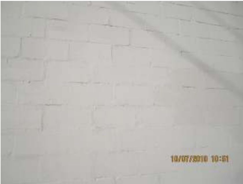
CMU repairs, typical
