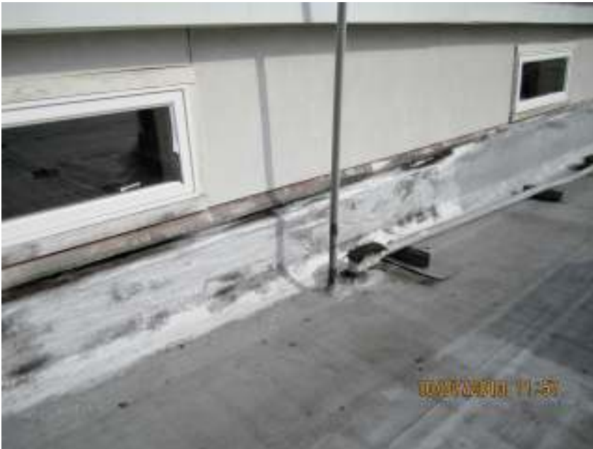
temporary roof repairs @ single drain opening
