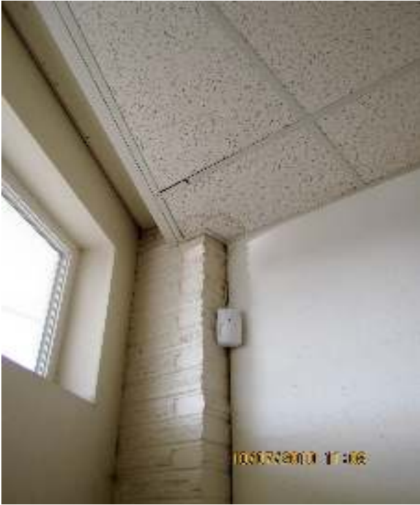
minor water damage @ SW corner
