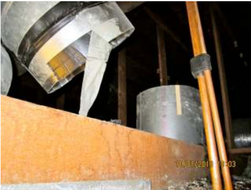
open attic duct work
