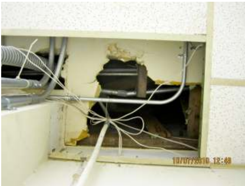
limited attic / drop ceiling view point
