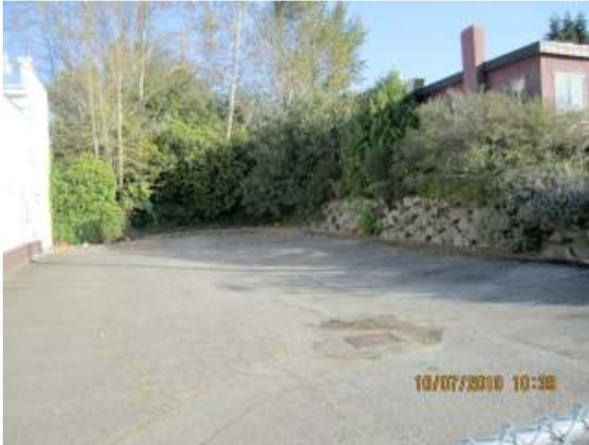
asphalt parking lot & catch basin
