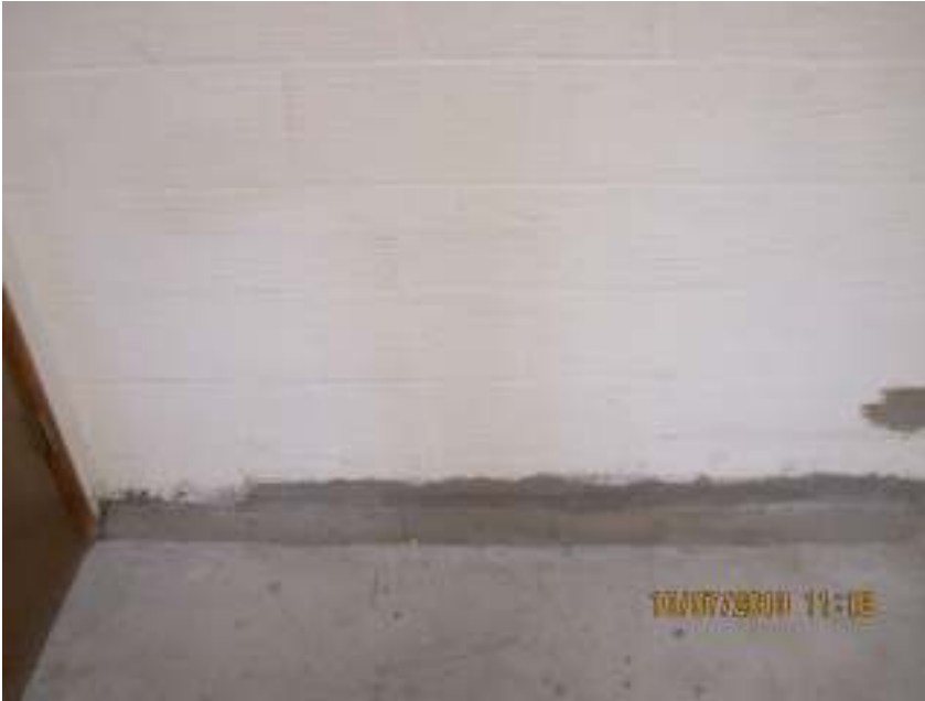
typical north wall water proofing
