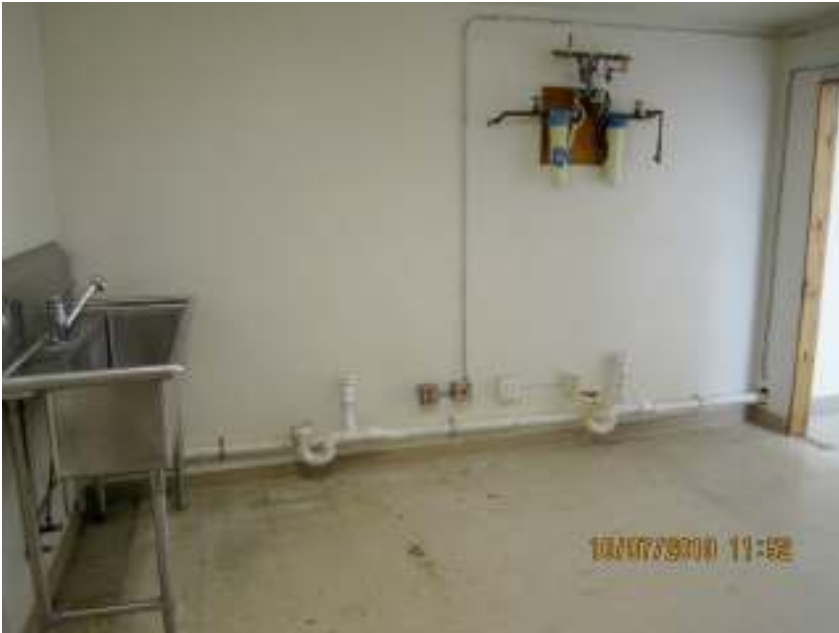
upper level wet room
