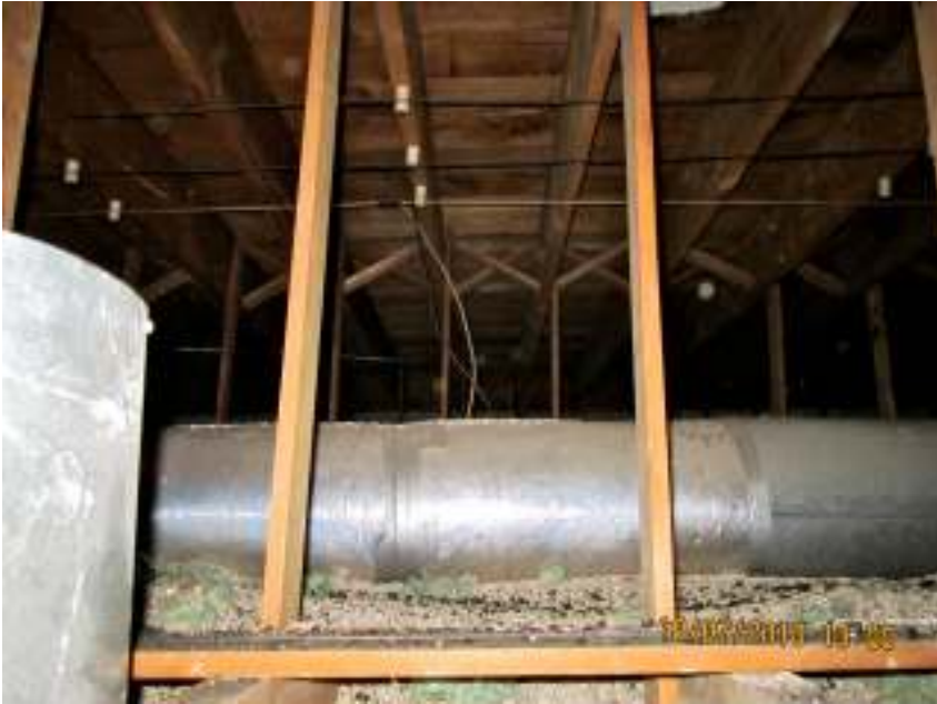
vermiculite office attic insulation
