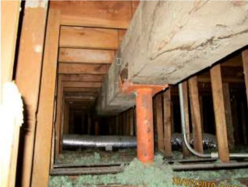
typical roof framing above drop ceiling
